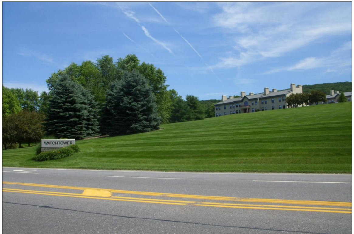
Looking northeast from Route 22 just south of Watchtower Drive. The southern portion of the Watchtower facility is shown, including one of the buildings associated with the Patterson Inn, an accommodation for guests of the Watchtower Education Center
