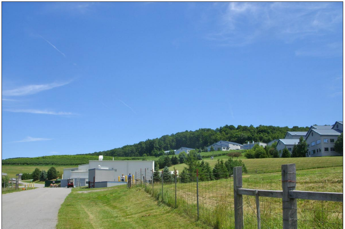
Looking northeast towards the concrete batch and recycling facility, from the northern portion of the road that diverges from the north side of Watchtower Drive. The orchard can be seen in the distance (left), as can several buildings within the northern portion of the south loop road (right) 6
