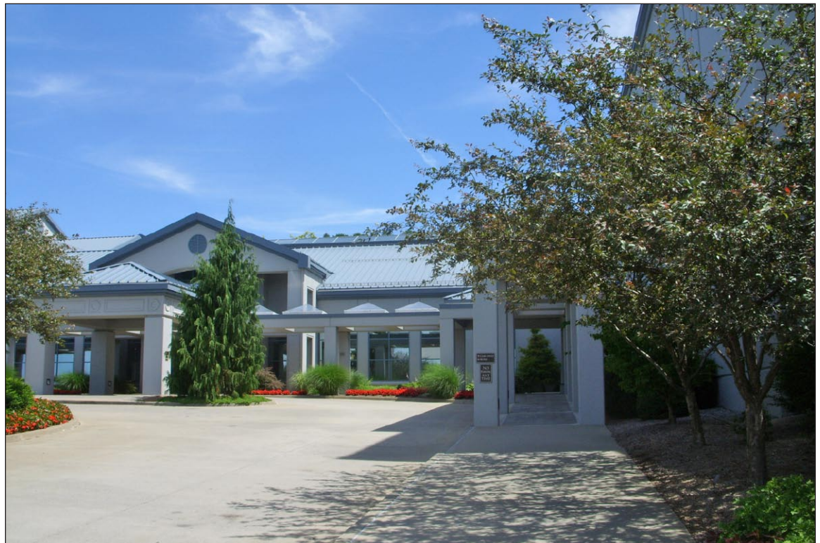
From the northeastern terminus of Watchtower Drive, a view looking north towards the entrance of the Main Lobby, contained within the loop road 4
